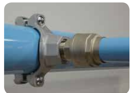
Attach Quick-Lock piping to fitting
